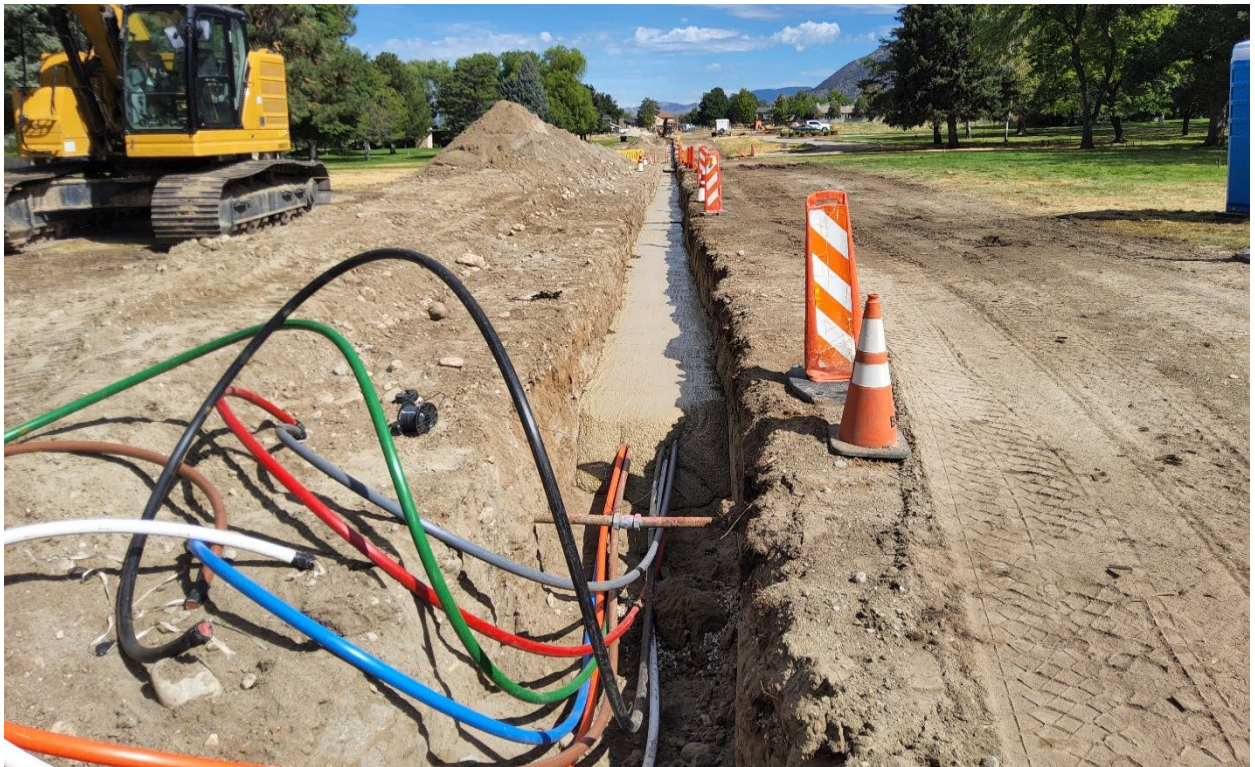
The fiber duct bank was installed through Memorial Estates above the SLAR.
