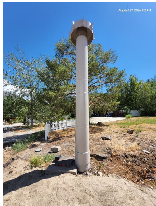
An SLA vent pipe was repaired and painted.
