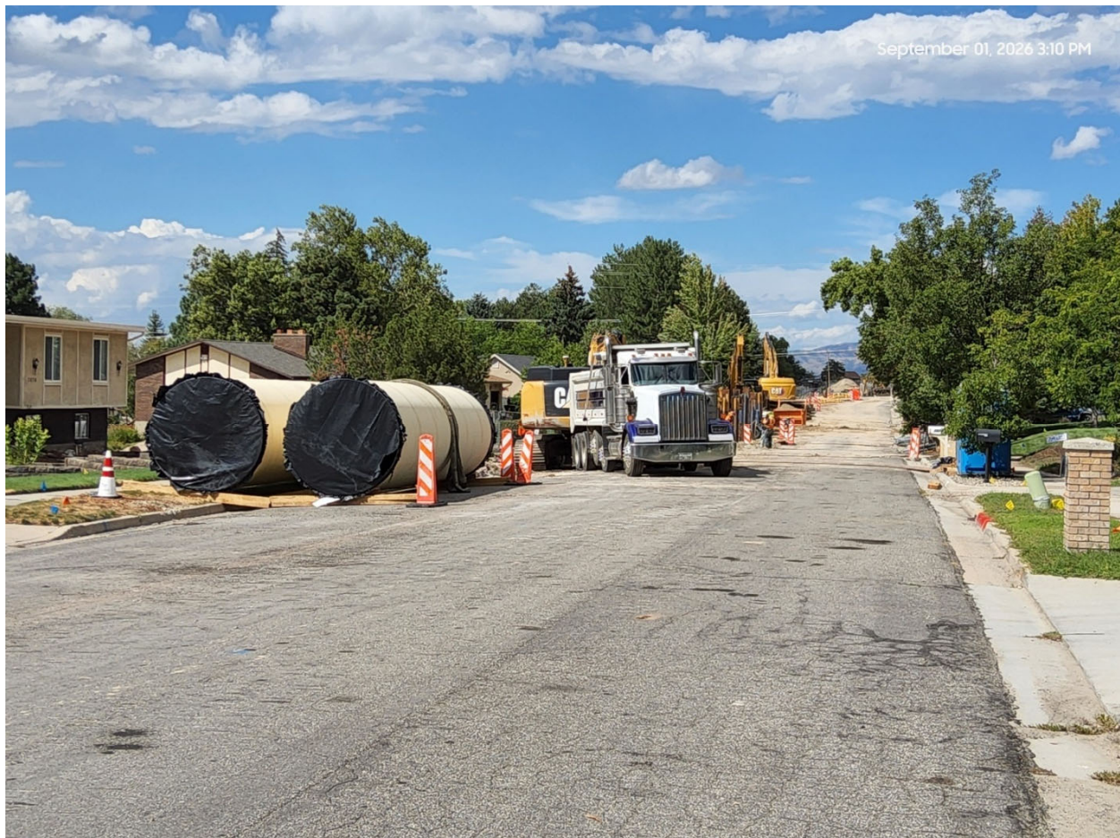
The SLAR is being installed in Deer Creek Road, south of Bengal Blvd.
