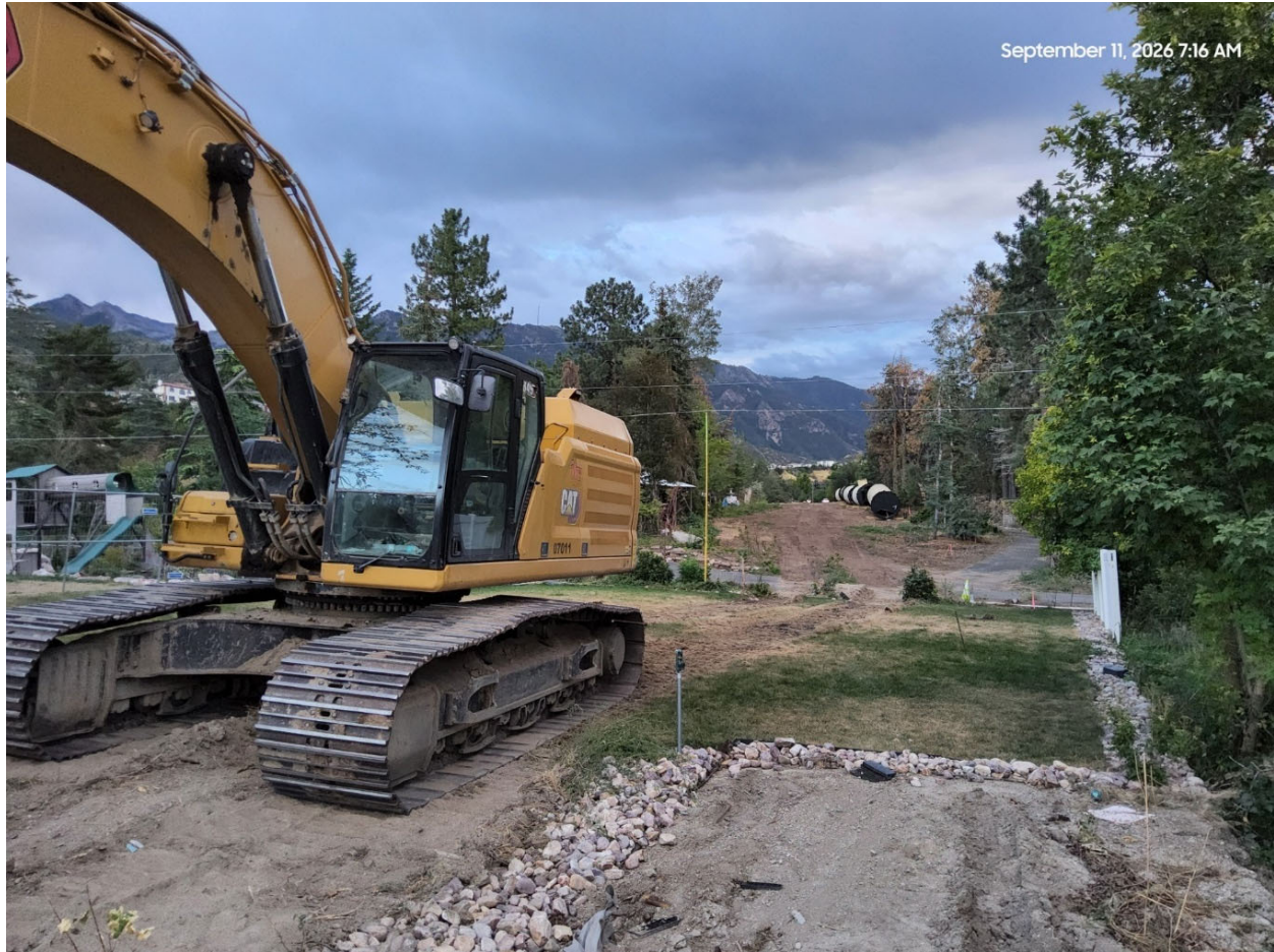
Installation of SLAR near Daneborg Drive on Danish Road.
