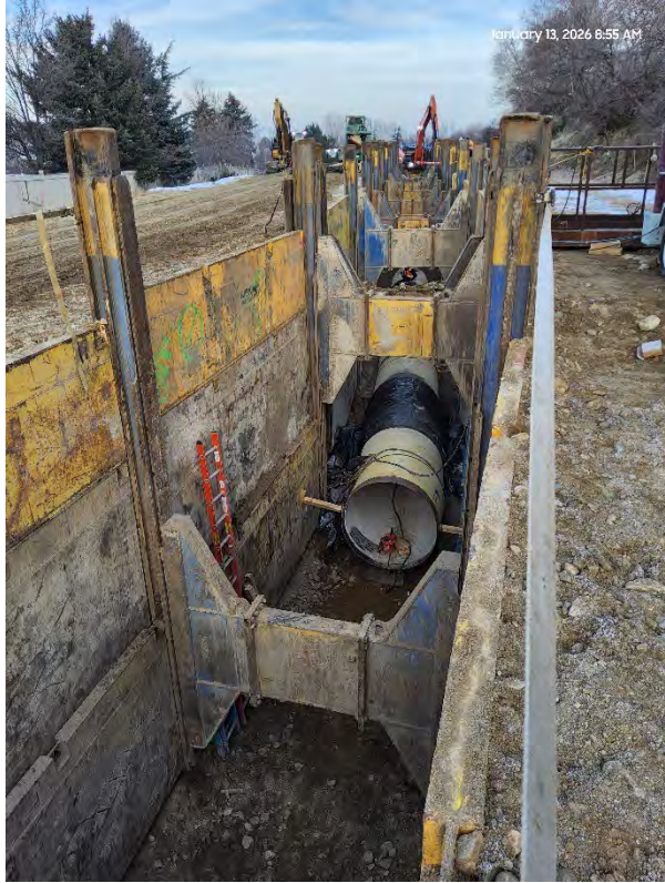
The replacement SLA is being installed in Danish Rd. The pipe will be connected in February.
