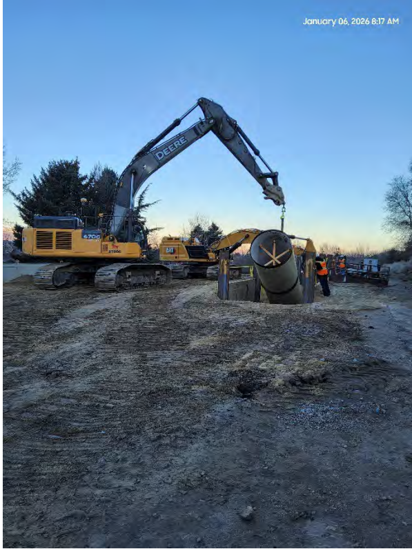
The replacement SLA is being installed in Danish Rd. The pipe will be connected in February.
