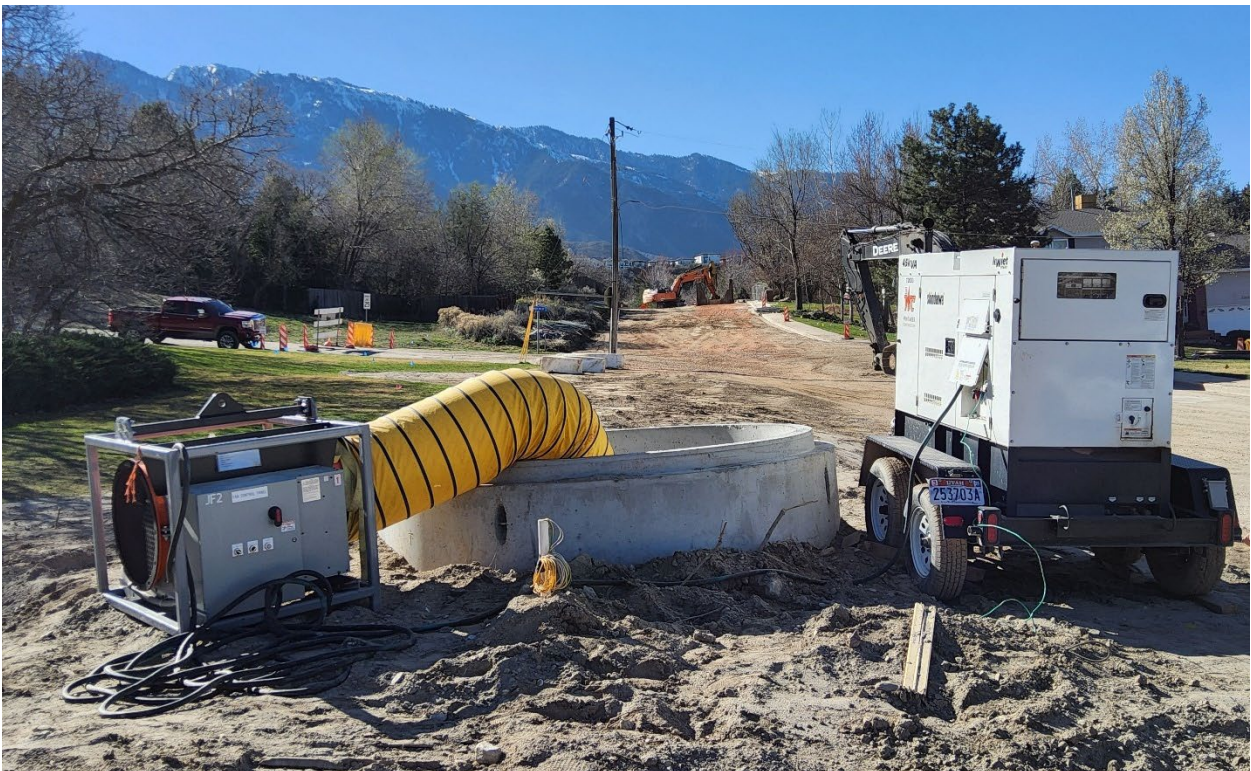
New Manway at Hidden Oaks Drive – Welding inside the Pipe
