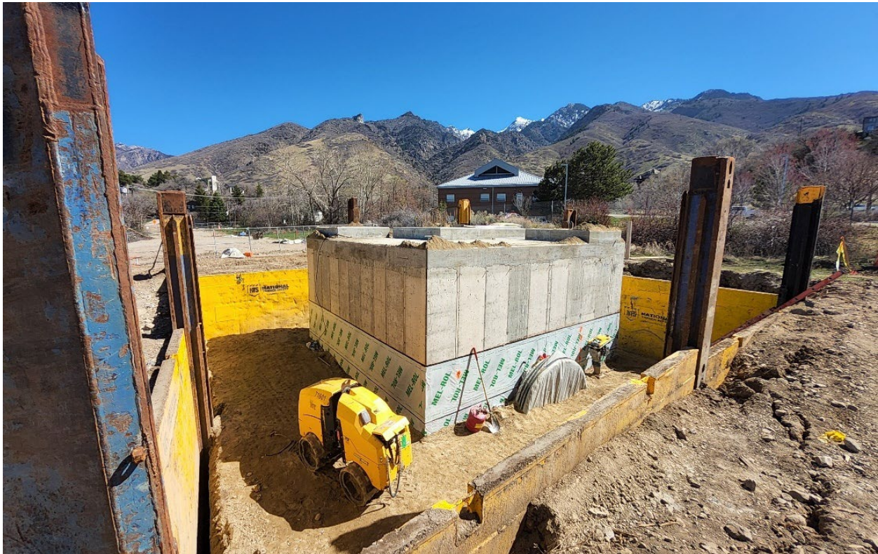
New SLAR Meter Vault – Ready for Backfill
