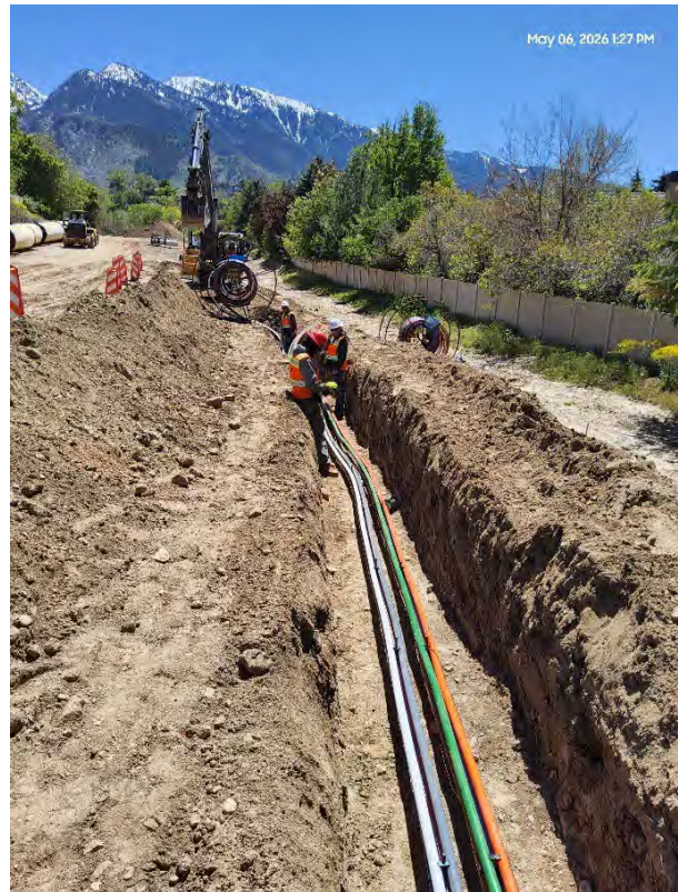
Fiber conduit install above SLAR in Danish Rd.
