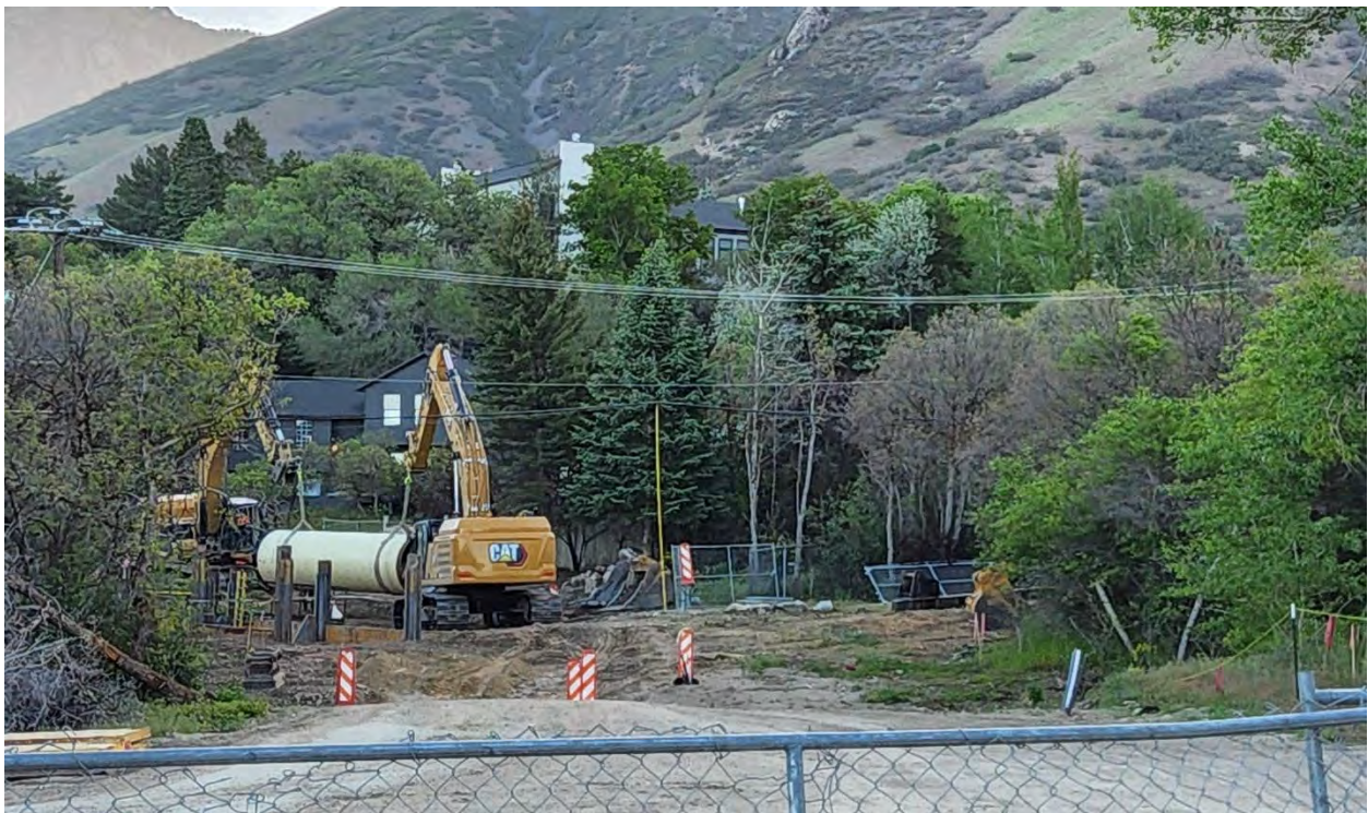
SLAR installation north of the Little Cottonwood Water Treatment Plant
