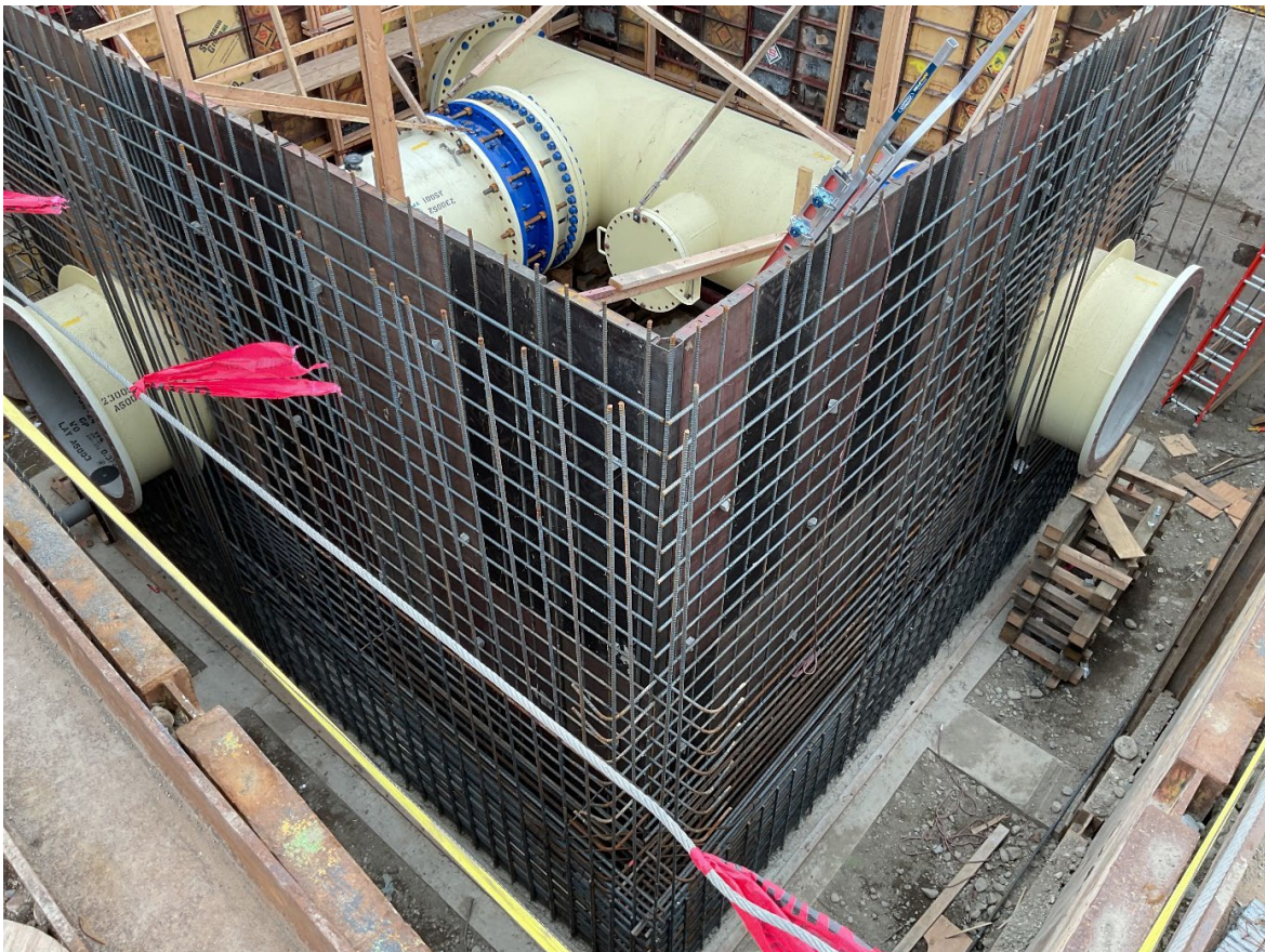
Feb 2: Rebar and forms for CC-1 vault walls is installed.
